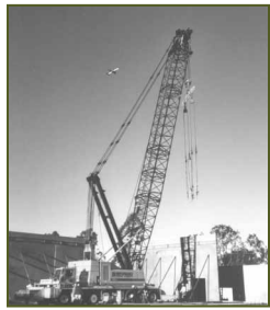
Bragg Crane Company tilting walls at Village of Hope
